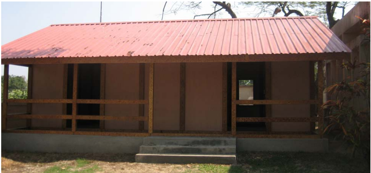
FABRICATED BAMBOO HUT
